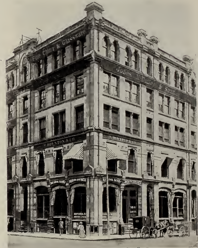
NATIONAL BANK OF NORTH AMERICA, 106 Franklin Street.
